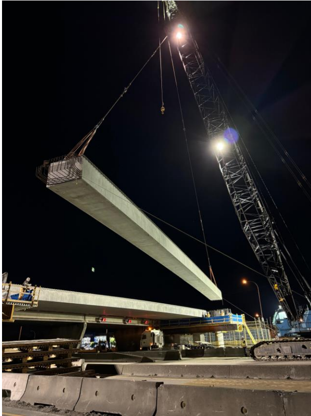
Heavy-lift crane hoisting a 35-metre, 50-tonne girder.
