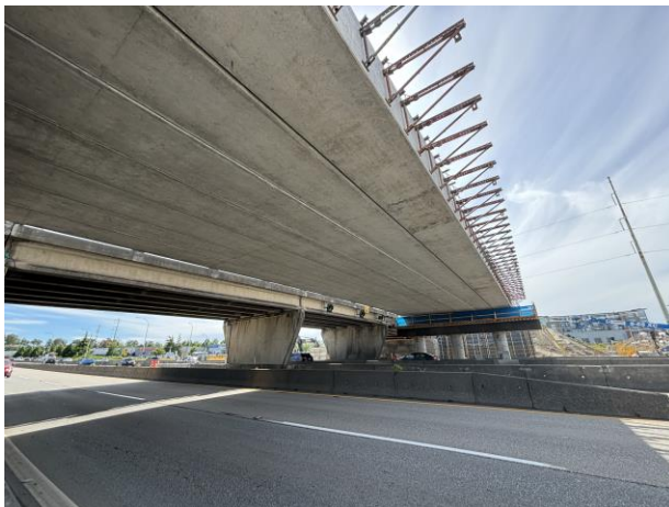
Newly installed Phase 1 girders spanning Highway 99.
