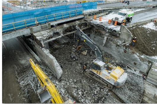
Excavators work to remove the east spans of the original Steveston Overpass (February 9, 2025)
